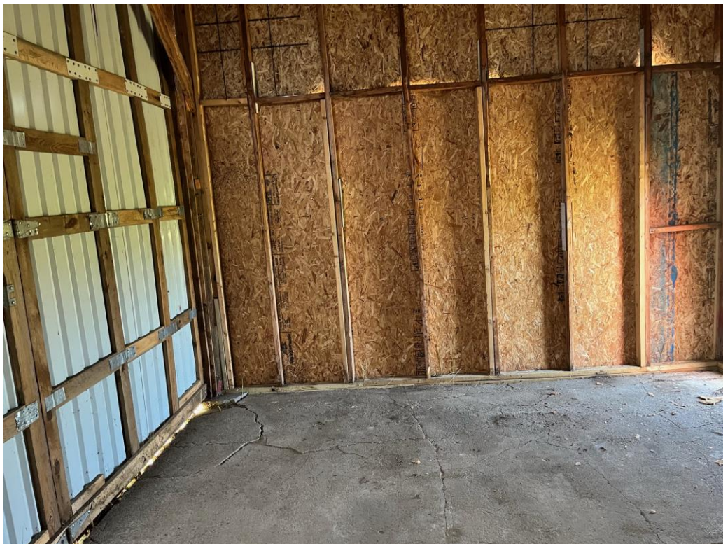
Interior view of one of the T-hangars showing the deteriorating concrete slab floor. Condition is similar in all three buildings. Image from 2024.
